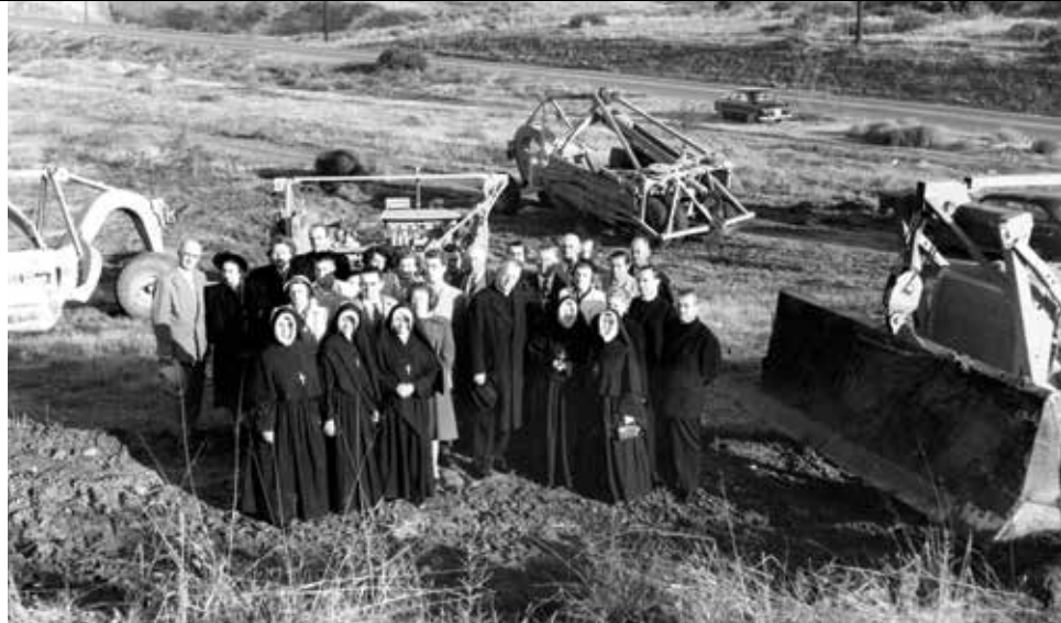
Groundbreaking at San Diego College for Women, 1949
