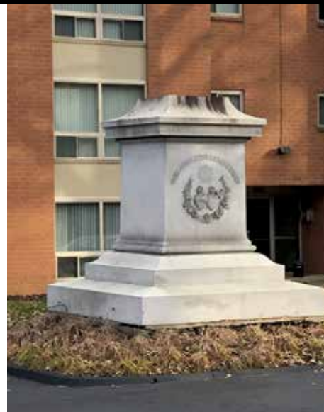
View of the pedestal at the West End Terrace Apartments before it was moved.
