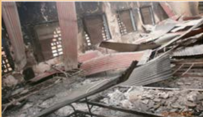
The dormitory that housed 200 students was completely destroyed.
